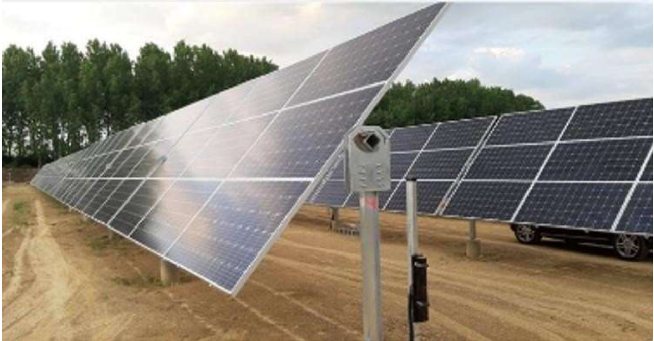
Figure 12: Tracking mechanism providing max 60° tilt angle to the north (i.e. about a fixed E-W axis)
