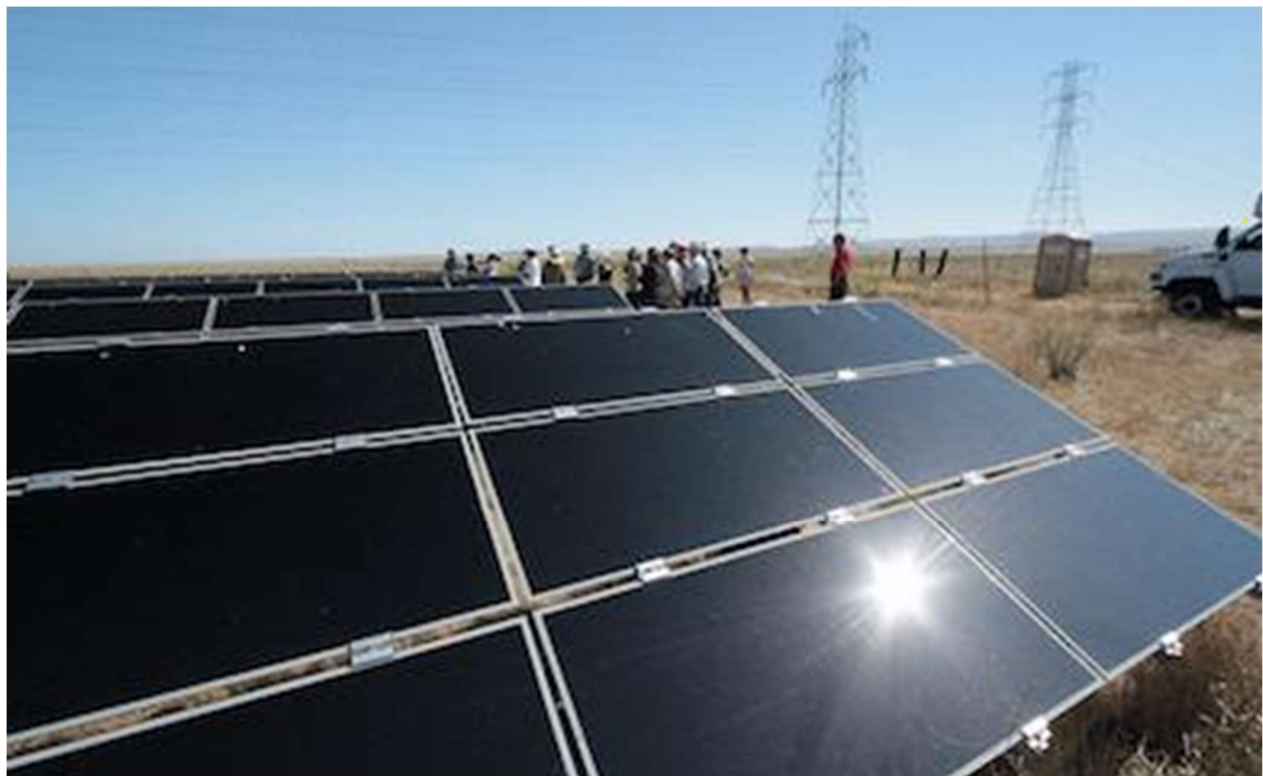
Figure 10: Typical PV module arrangement in N-facing frame, with variable tilt about the E-W axis
